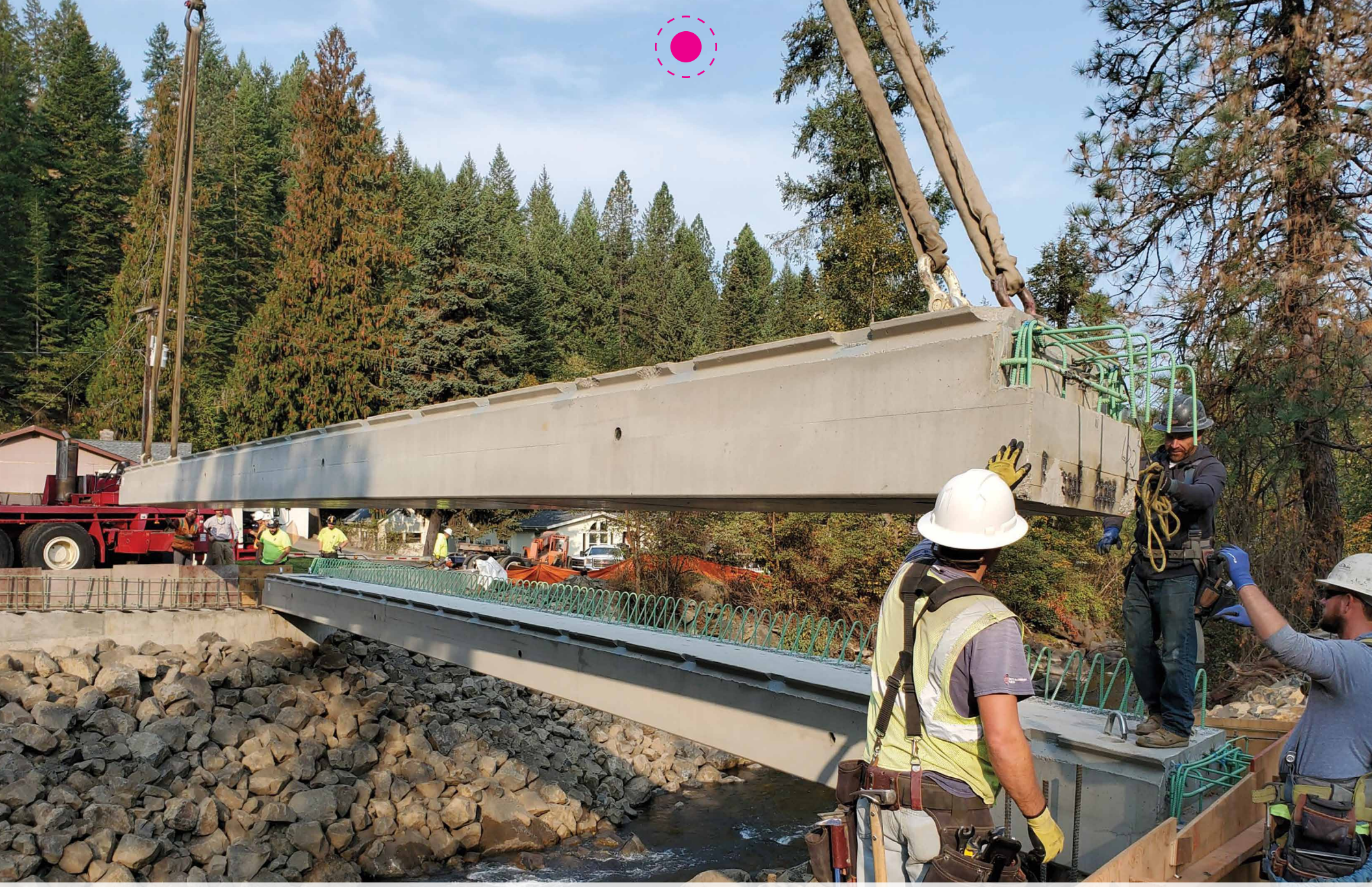
Mike Slegers, HDR Orofino Creek Bridge Construction
