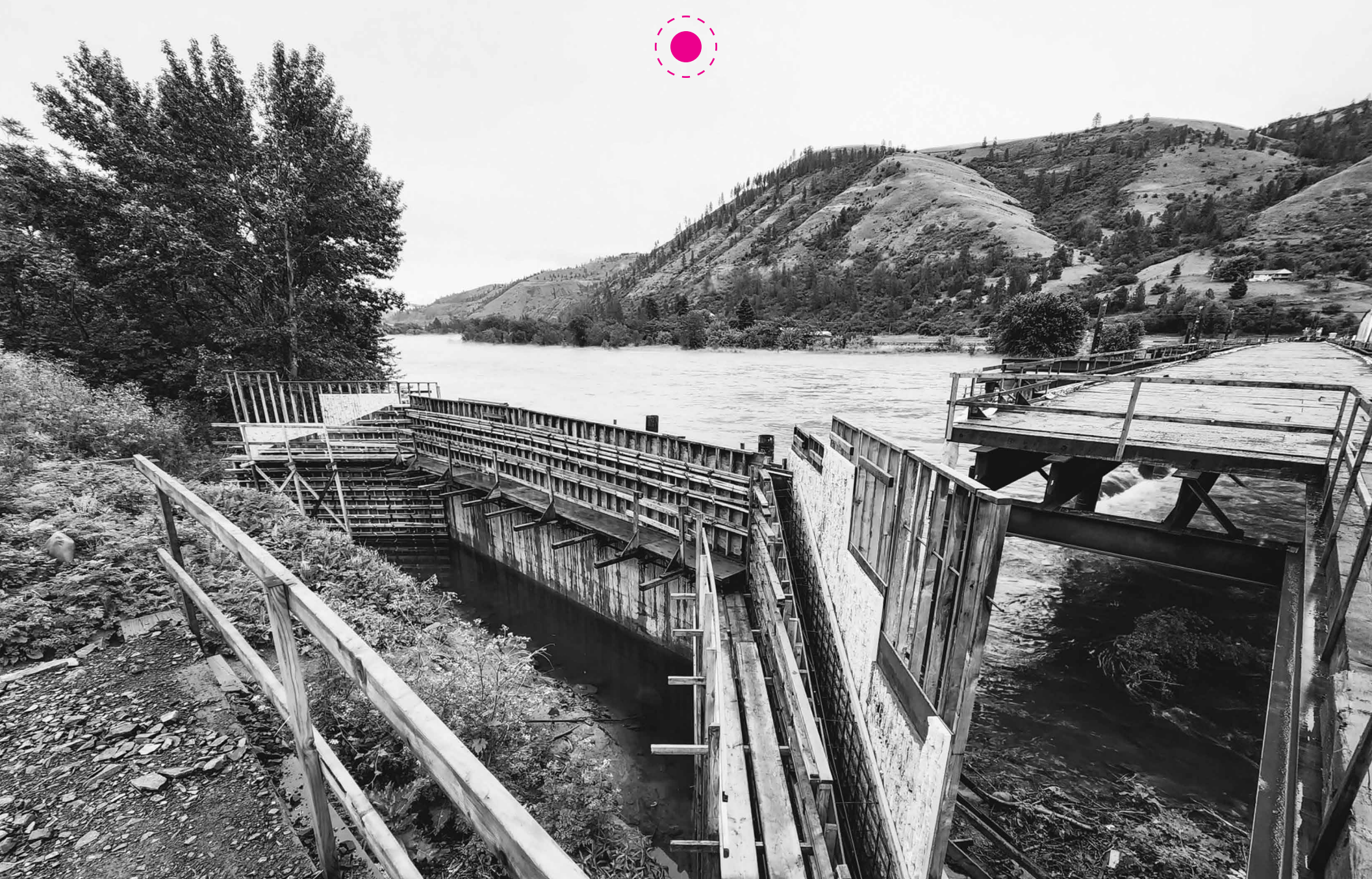
Jake Southwick, Civil Science Inc. Cherrylane Bridge Construction
