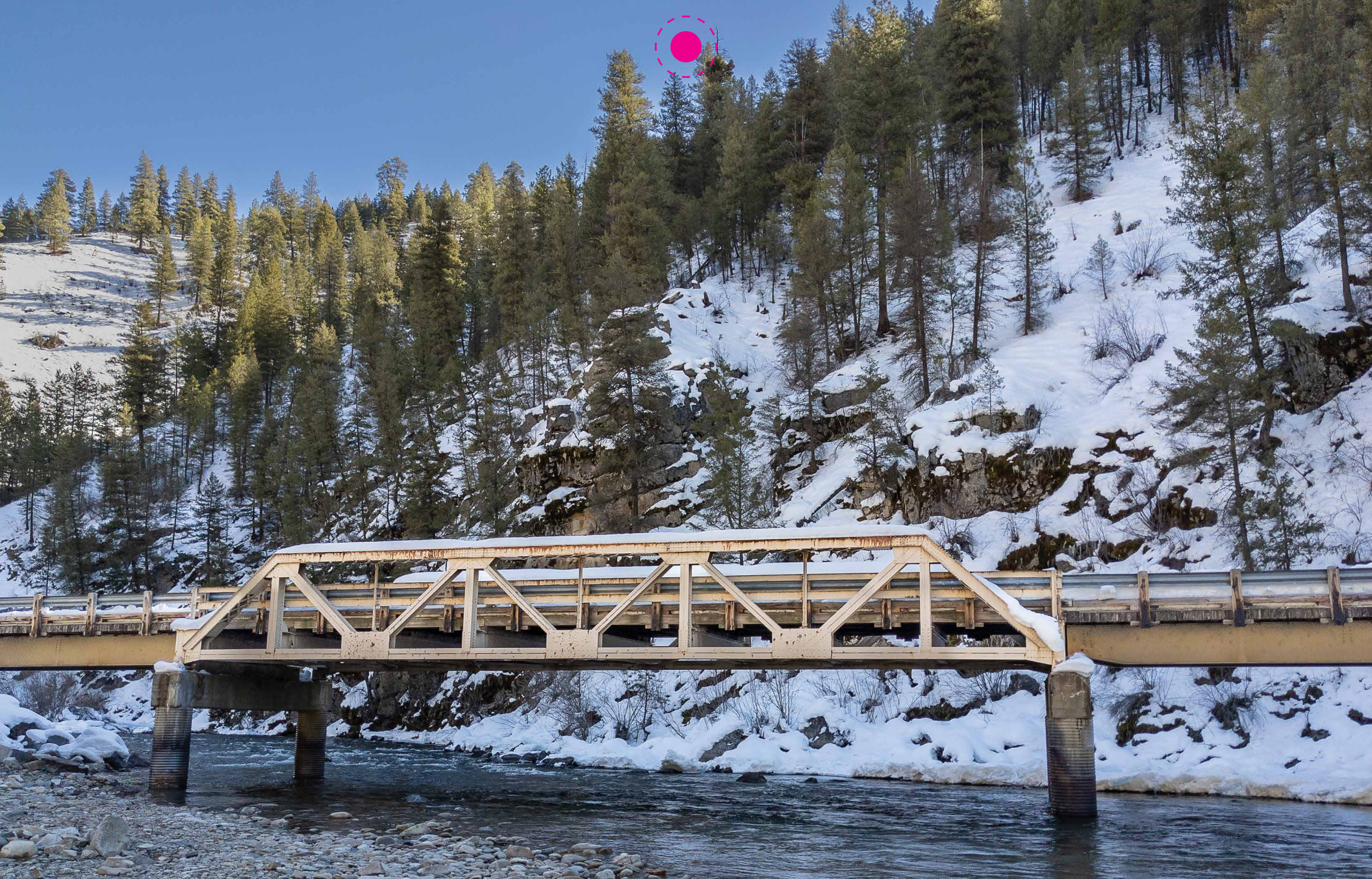
Jake Melder, LHTAC Arrowrock Road Bridge Over the MF Boise River
