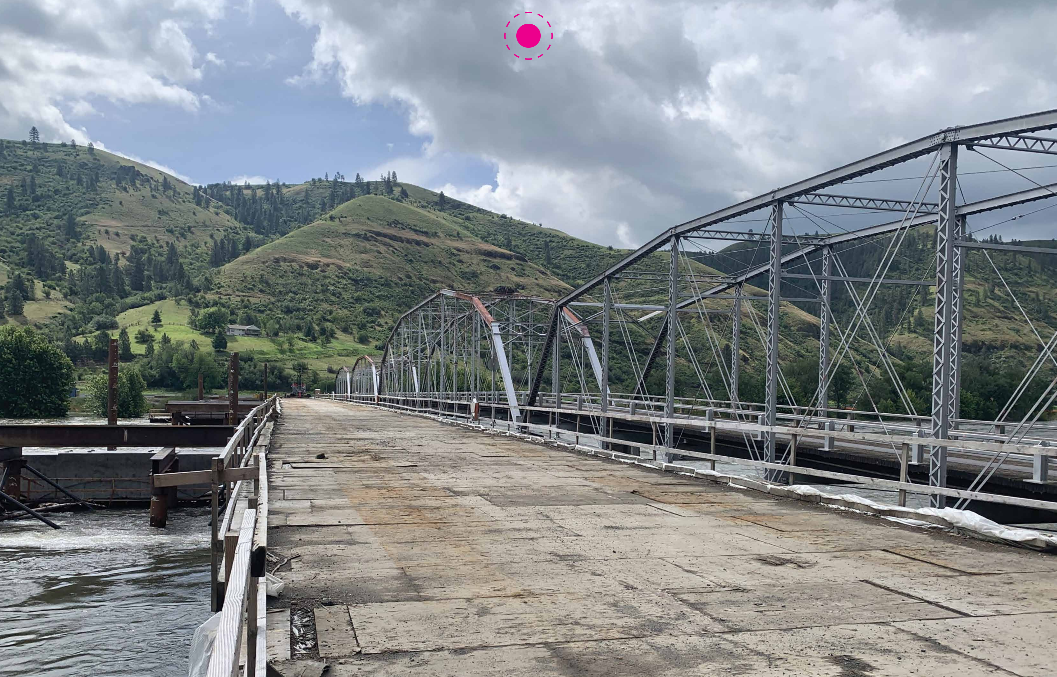
Karissa Nelson, LHTAC Temporary Bridge on Cherrlyane Bridge Replacement
