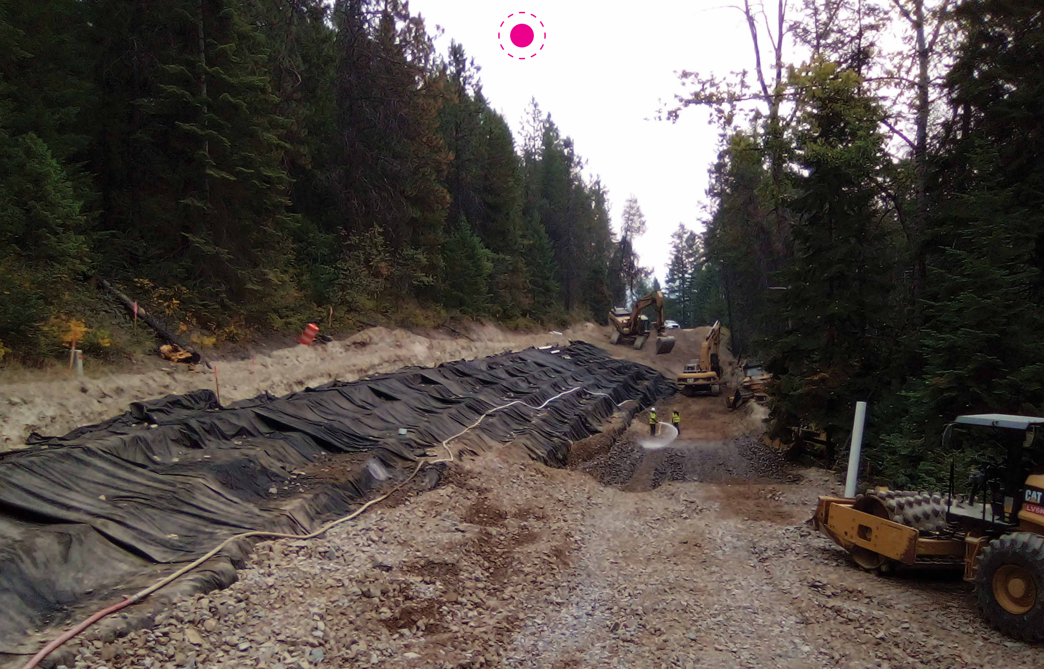
Jeffrey Spohn, DEA Inc. East River Road Repairs Bonner County
