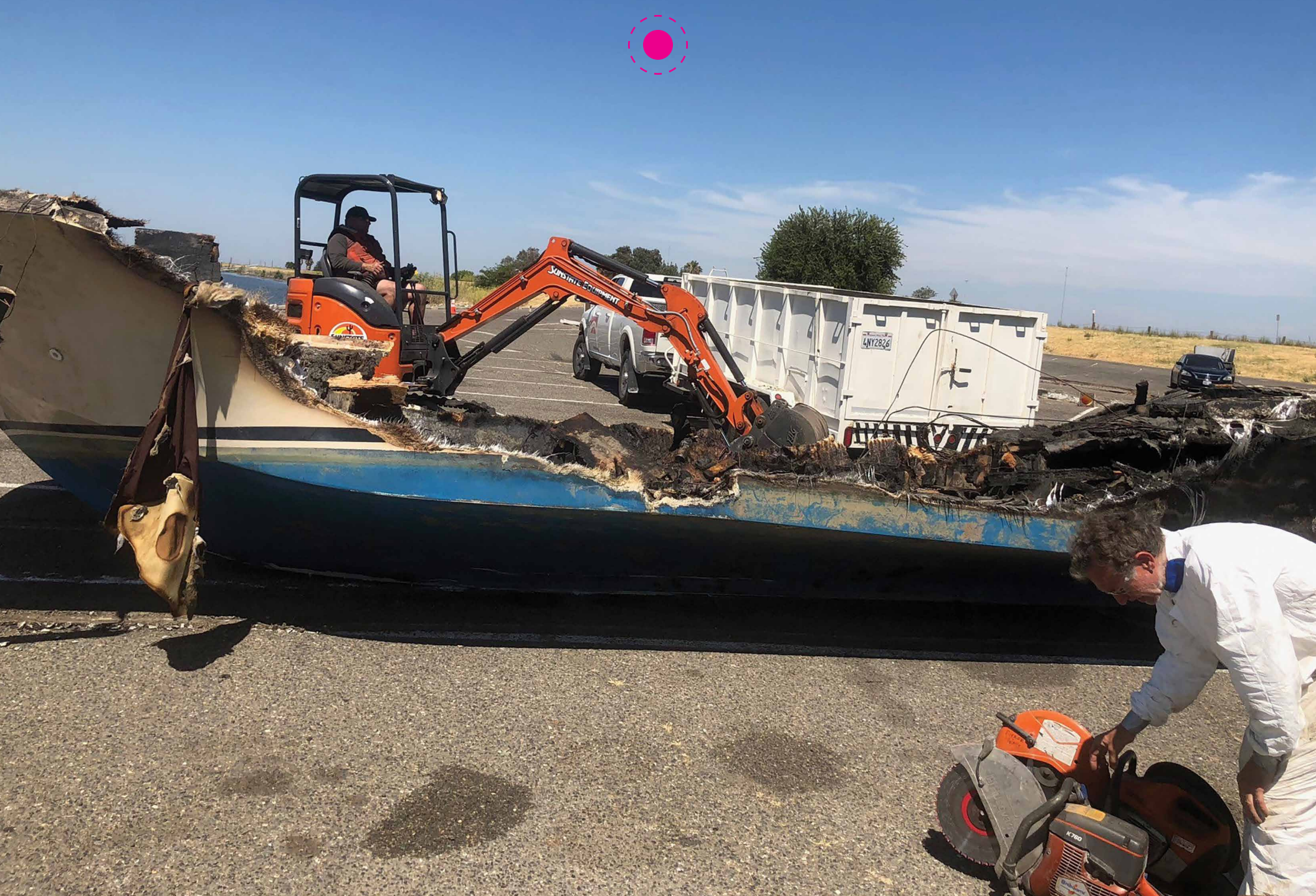
PDS crew raises, tows, then disposes of 36’ houseboat that burned, capsized, and sunk in the Sacramento River.
