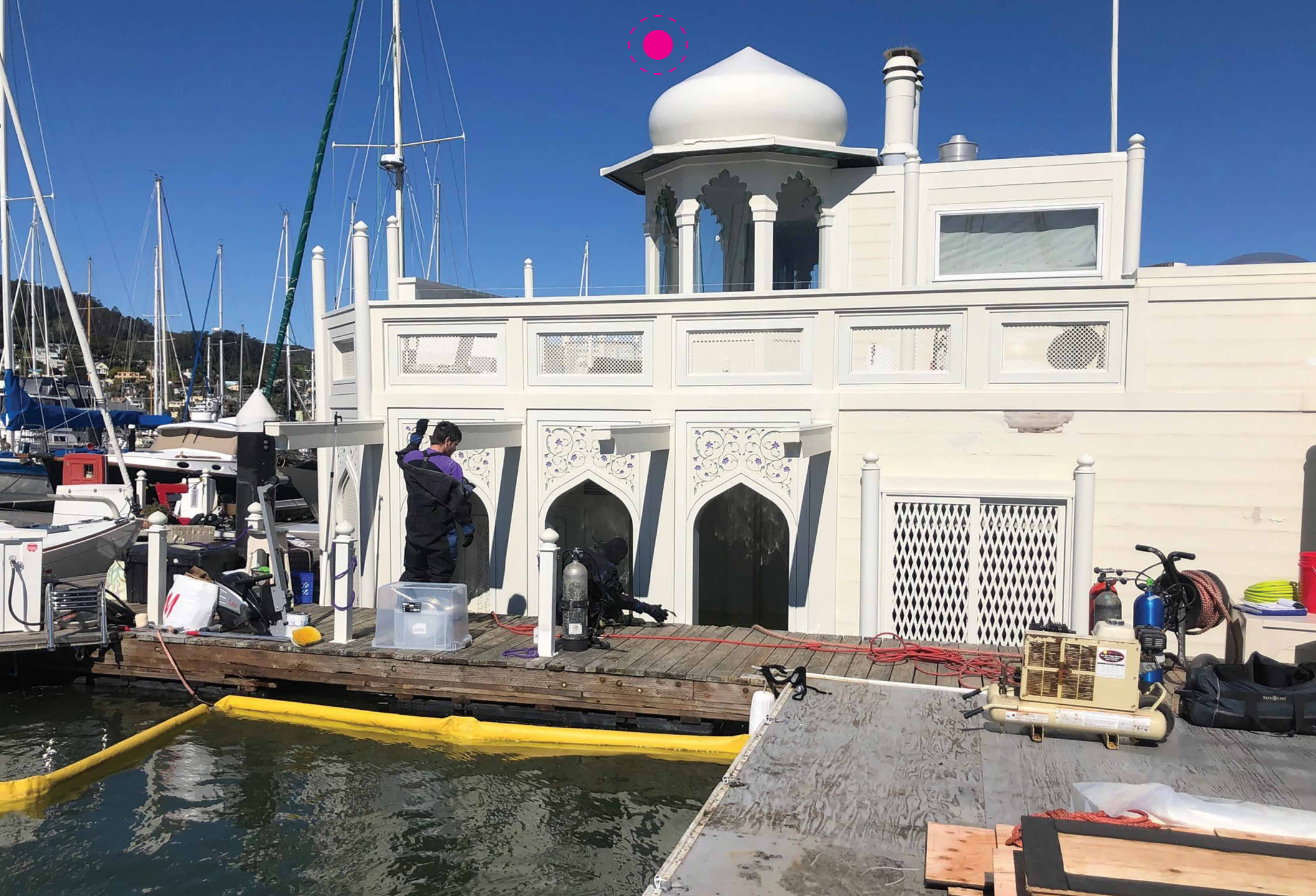
The famous floating home “Taj Mahal” sinks during the unprecedented bomb cyclone in the Bay Area.
