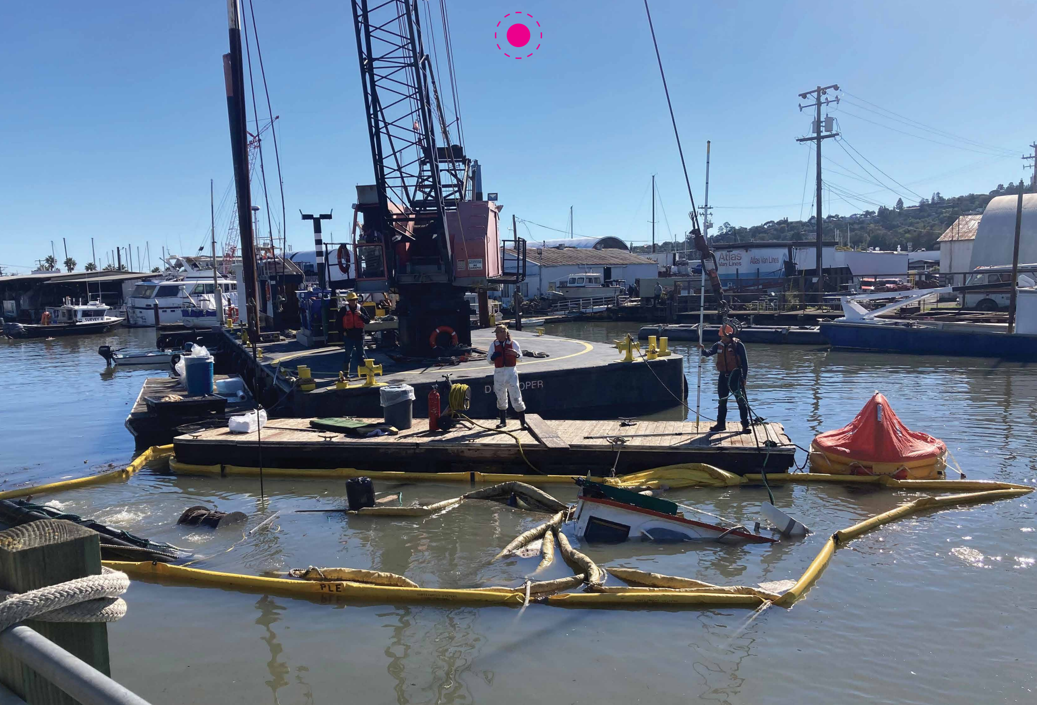
San Rafael Yacht Harbor’s crane and PDS divers chip in to raise the 42’ Steel Tug, “R.H. Percy” sunk in San Rafael Canal.
