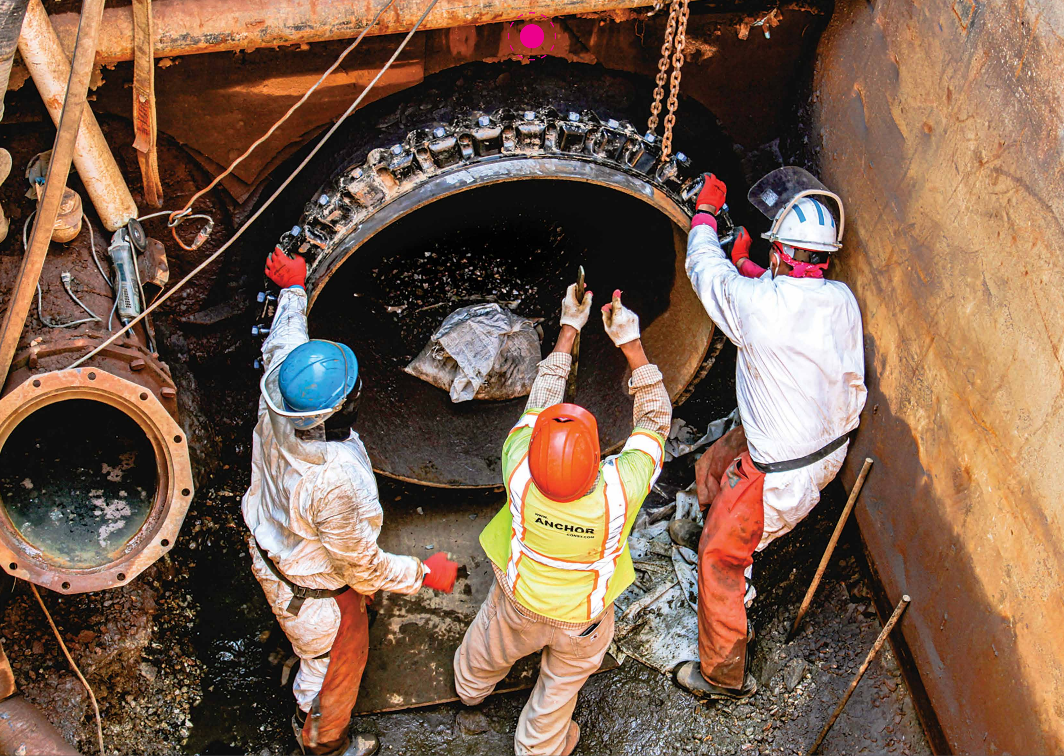
Anchor Unit 32 replaces aging infrastructure in the City of Baltimore.
