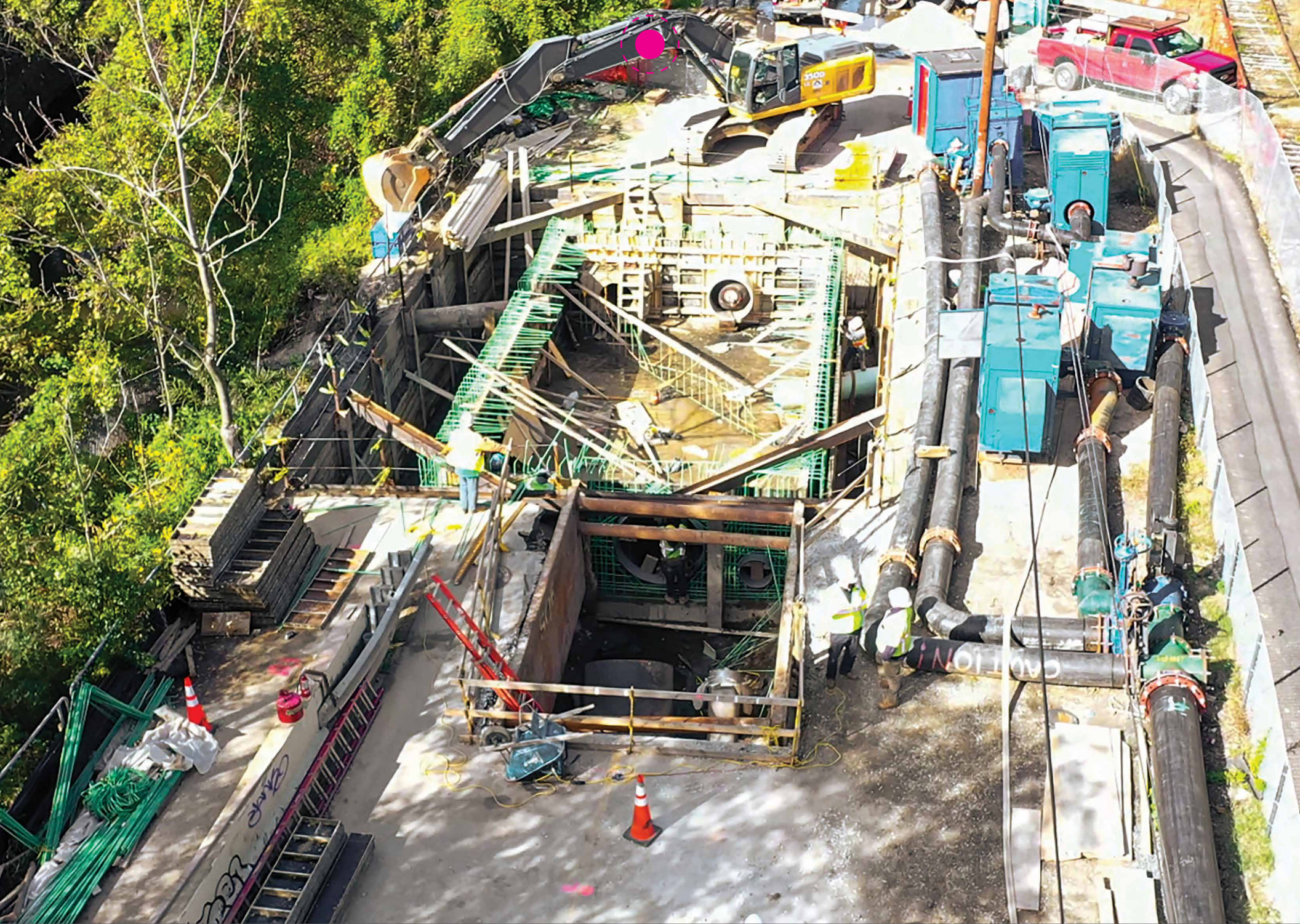
Anchor Unit 32 replaces and rehabilitates thousands of linear feet of sewer main in the City of Baltimore.
