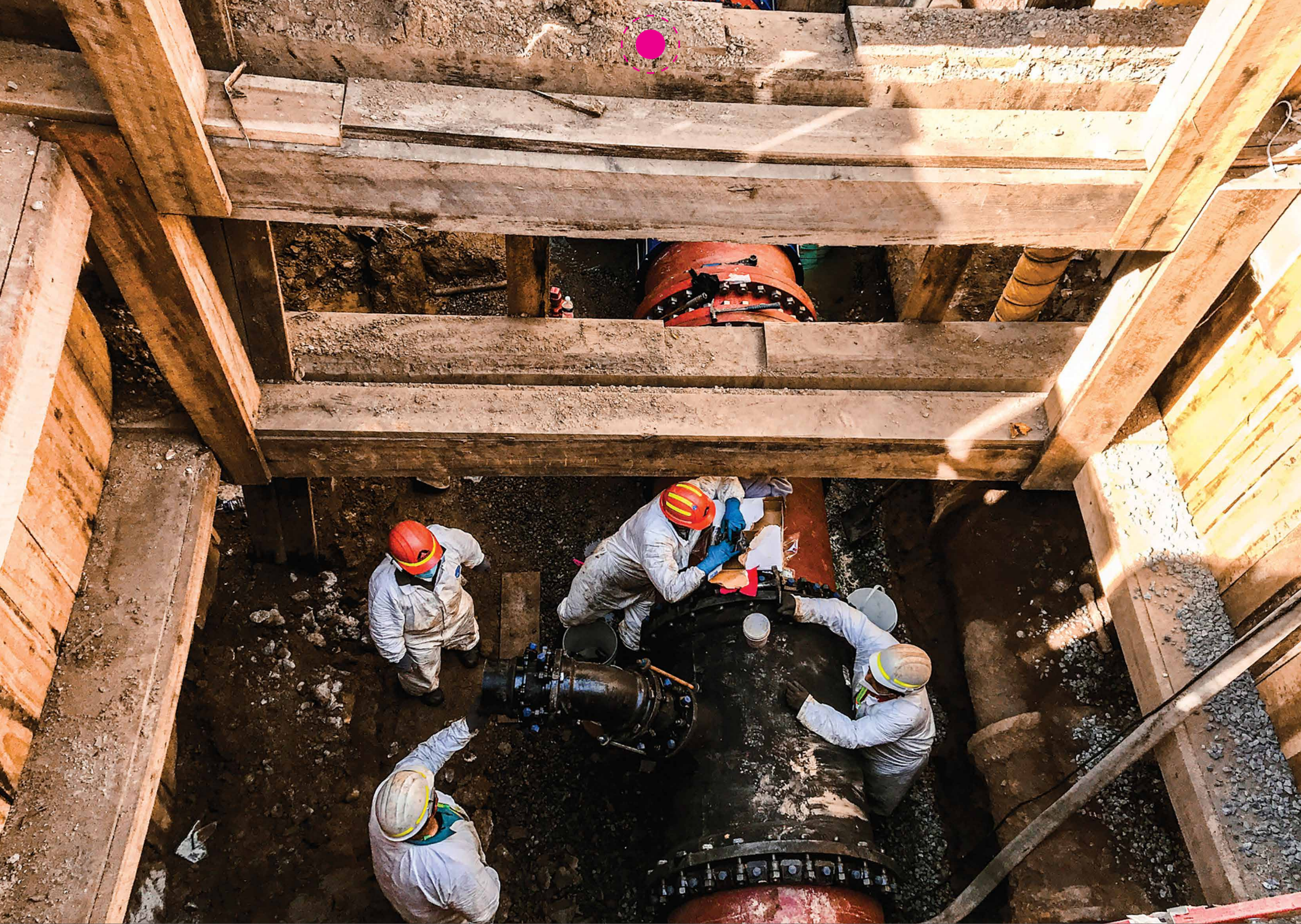
Anchor Unit 29 completes repairing a large valve for DC Water.
