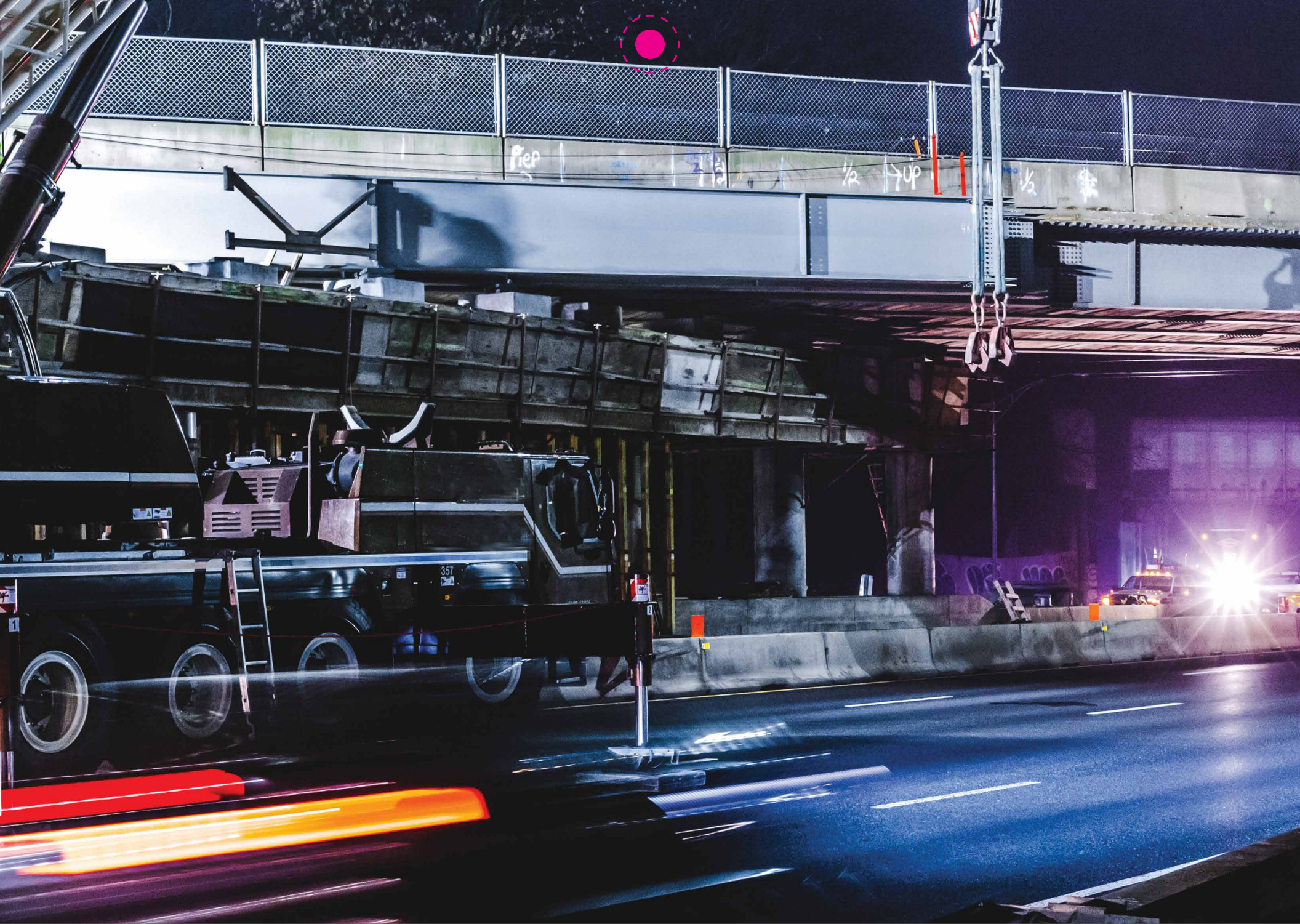
Anchor Units 49, 84 & 40 completes a beam placement on the MDOT-SHA Seminary Road Bridge project.
